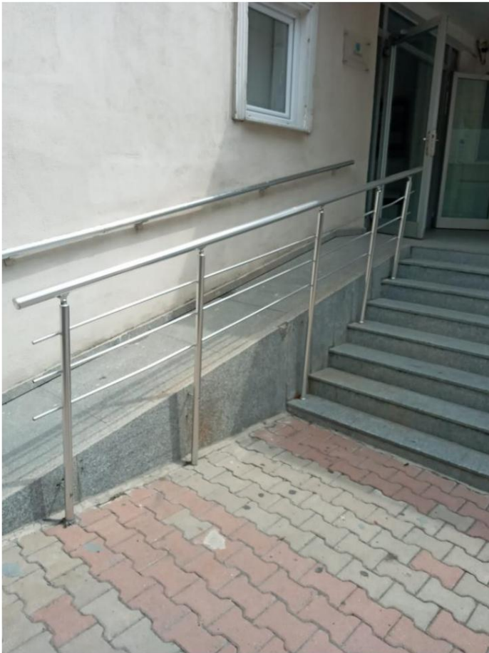
Disabled ramp at the entrance of Block F
