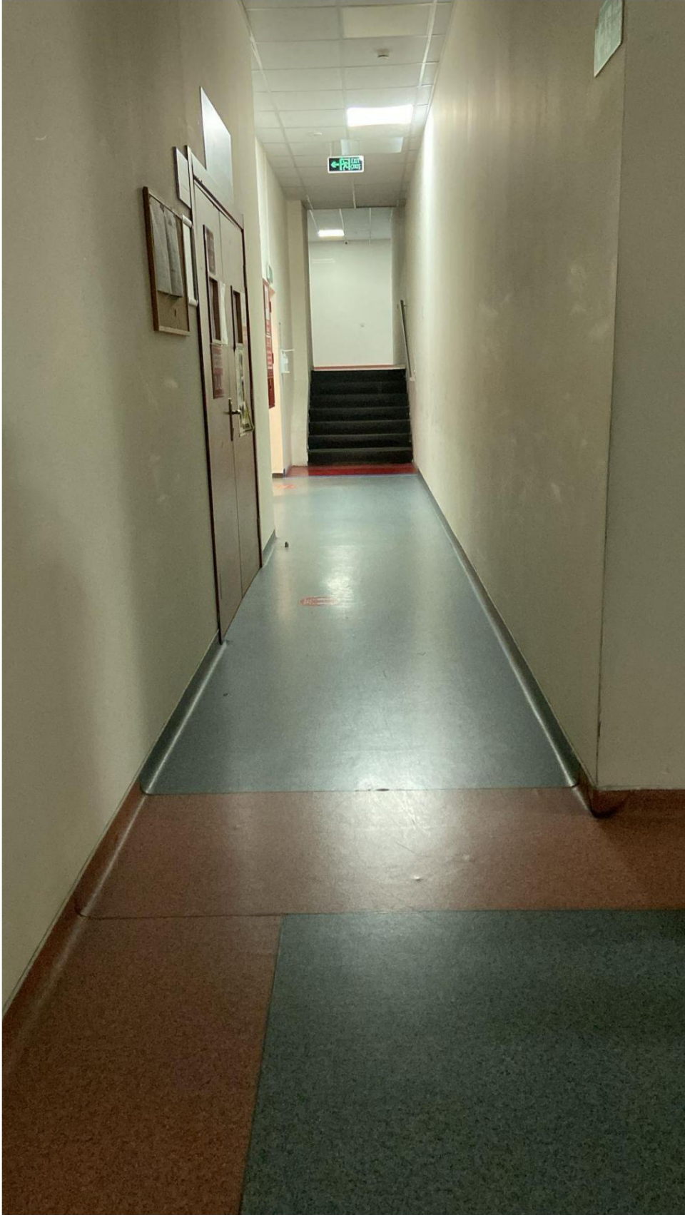
Library entrance door in Vocational School Building (left)
