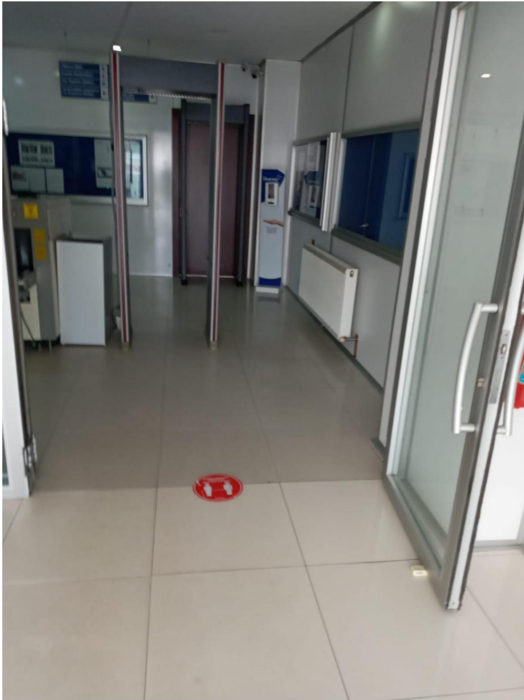
A view from the step-free floor at the entrance of the building
