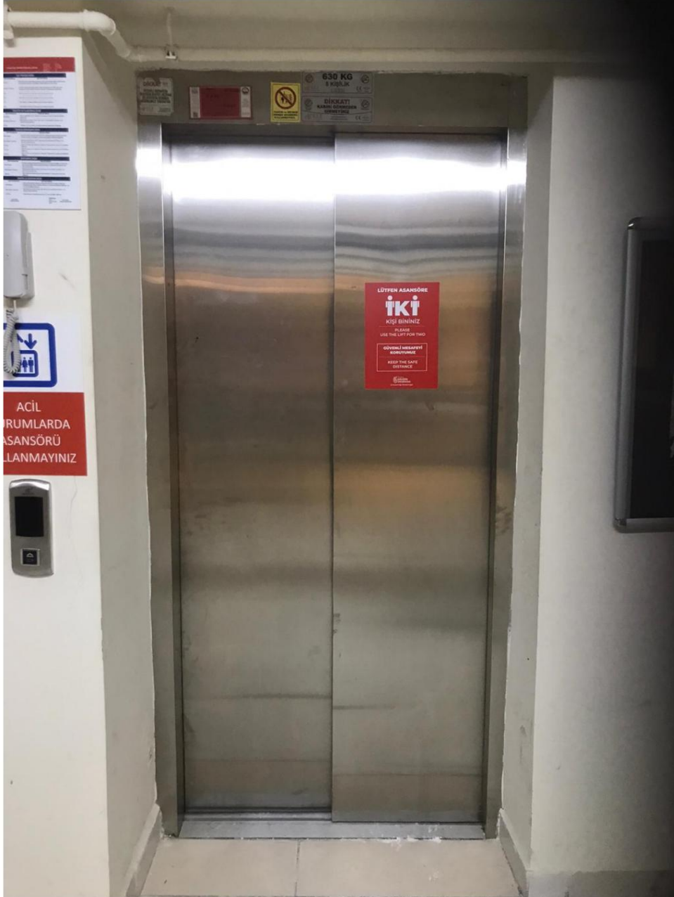
Building entrance and elevator
