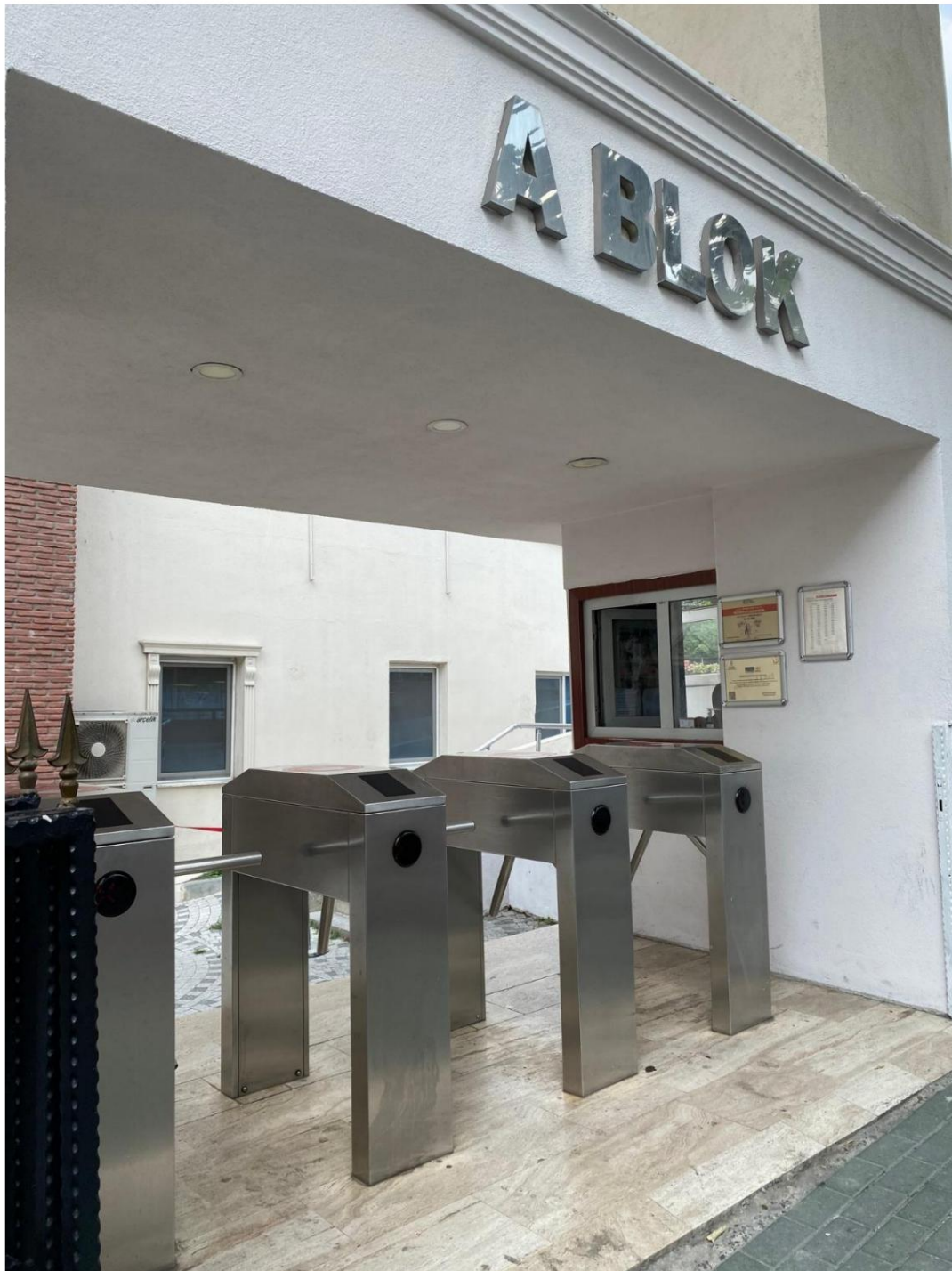
Block A entrance
