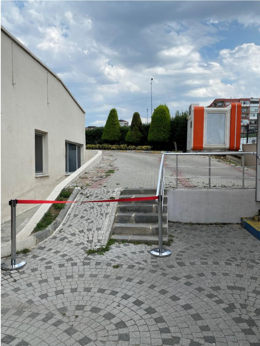
Block A ground floor transition ramp
