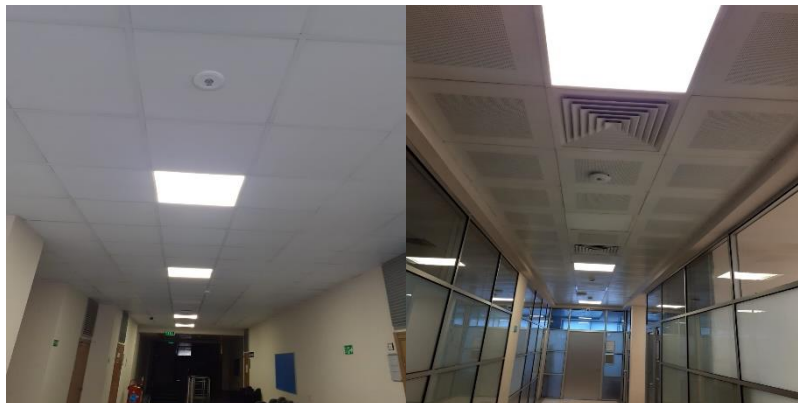
Figure 1. Some areas of Block G with lighting works
